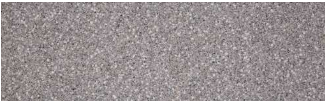
A-403 Asphalt Material
